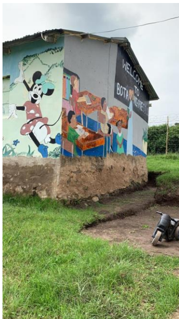
Figure 2 Outside Botani ECD school. Note the illustrations on the wall but base of building is losing plaster therefore subject to damp.
